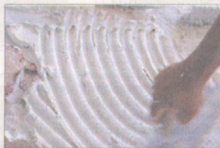
AndersonSargent Custom Builder's entry in the annual home show gets stonework inside.
